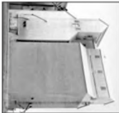
2. Metal-clad elevator with metal-clad annex.
